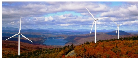
Renewable Energy Vermont
